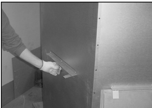
Figure 4.6 Bending Refractory Shipping Tabs Back Down
